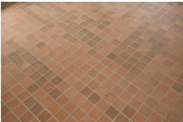
Items are named after the size of the mold in which they are produced. The tiles will invariably shrink during the drying and burning process.
